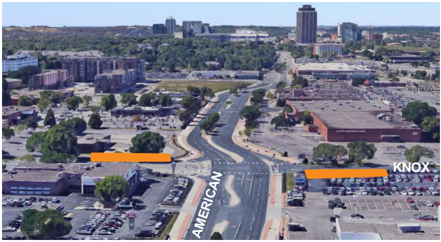
American Boulevard Station
