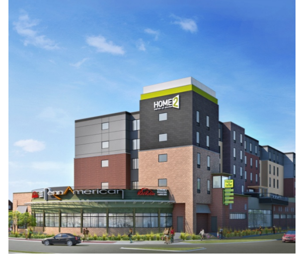
Adjacent TOD (under construction)
