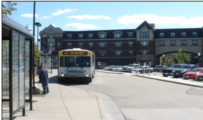
46 th St LRT Station, Minneapolis
