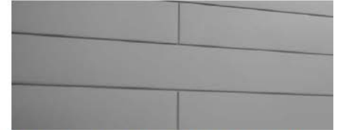
Station Cladding - Metal Panel
