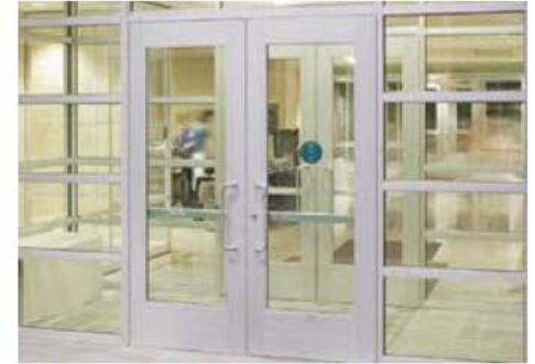
Entry - Metal & Glass Doors
