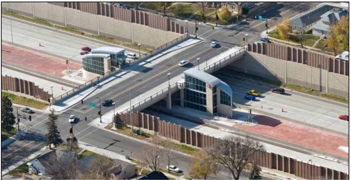
Figure 10. Aerial View of 46th Street Station
