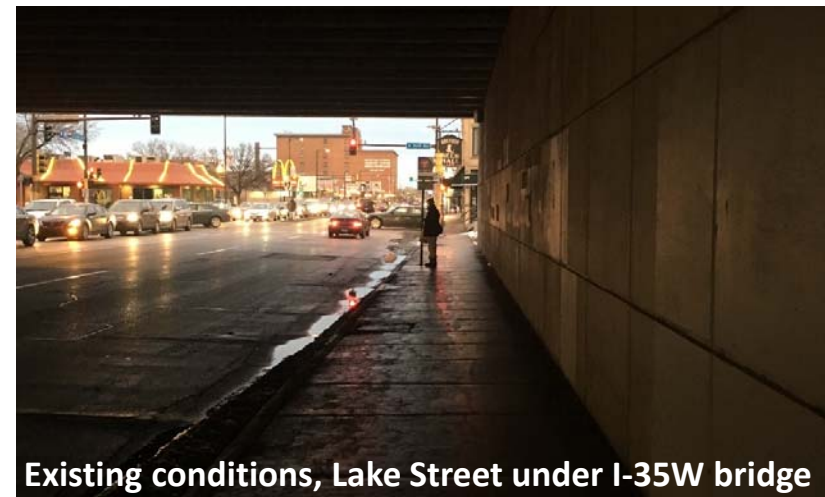
Existing conditions, I-35W at Lake Street
