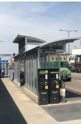
Platform Shelter (A-Line shown)
