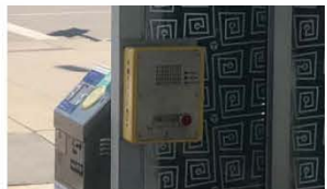
Emergency Telephone (A-Line shown)
