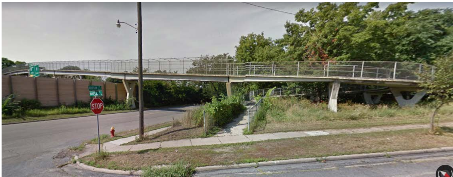
Maple Street Pedestrian Helix and Bridge over Hudson Road and I-94
