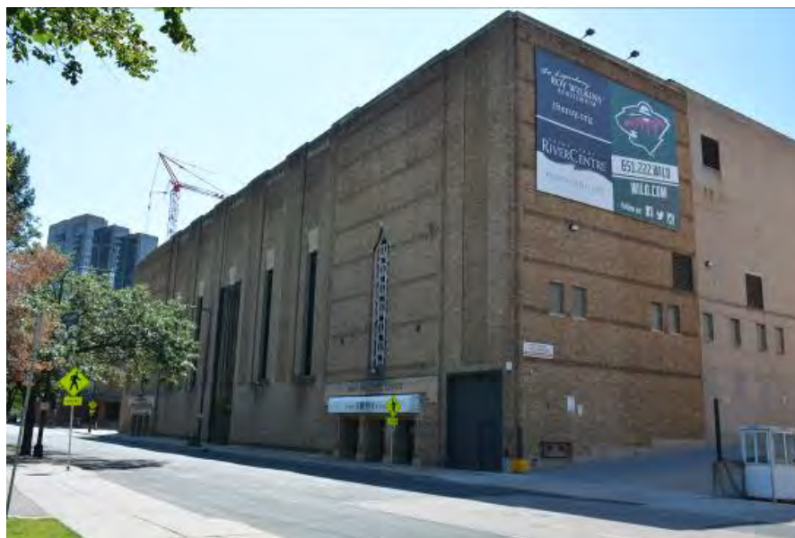
Figure 69. Saint Paul Auditorium Addition, facing east
