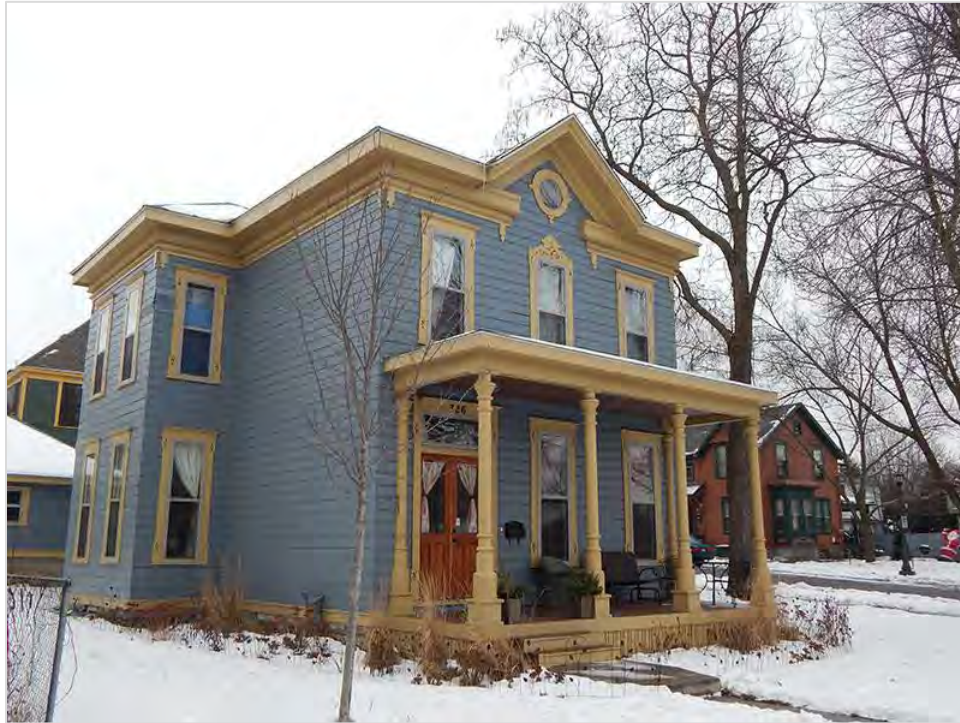
Figure 29. Peter Bott House, facing east
