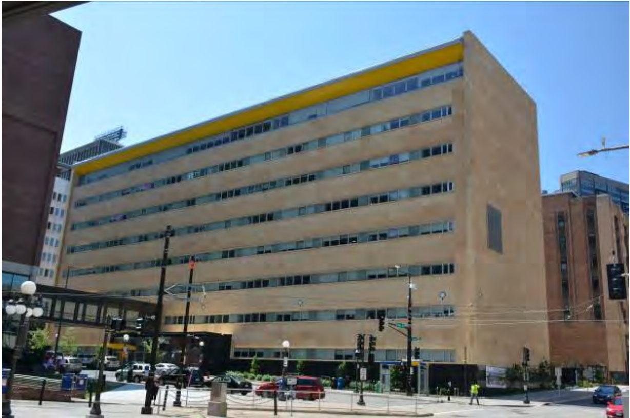
Figure 55. MMLI Building, facing south
