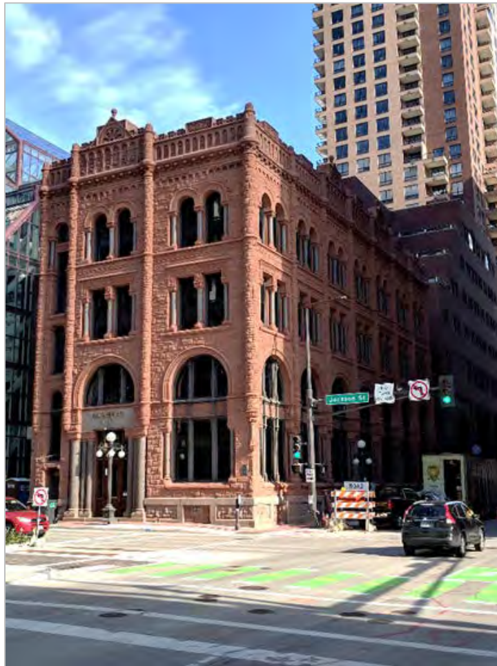
Figure 42. Merchants National Bank, facing northeast
