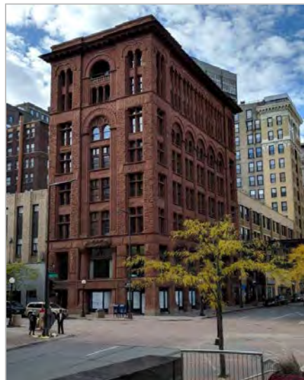
Figure 57. Germania Bank Building, facing southwest
