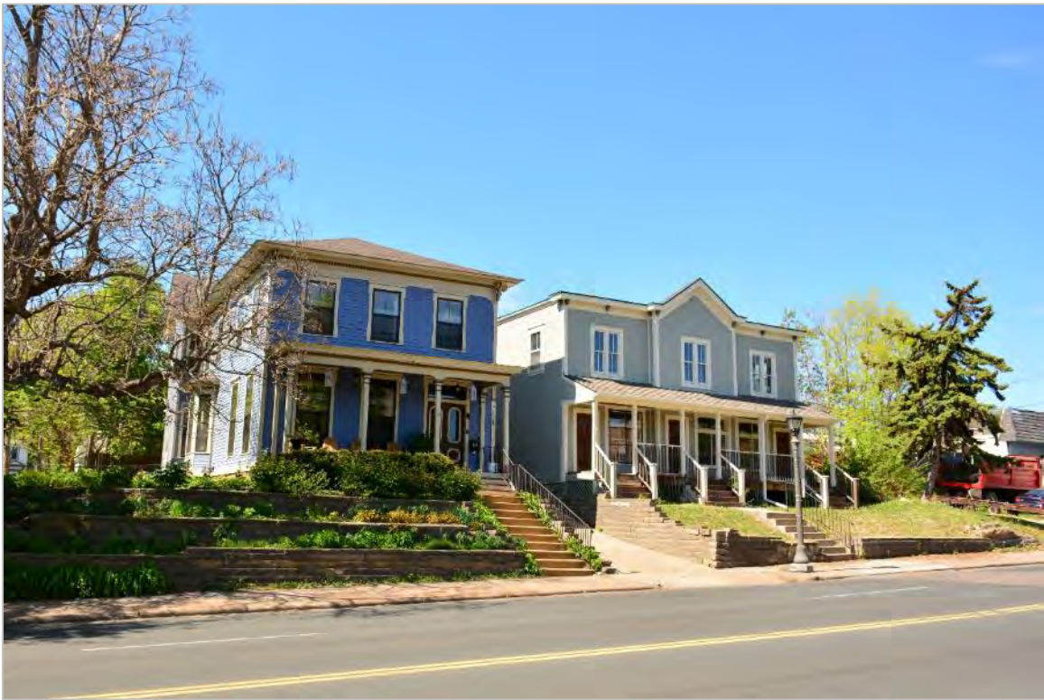
Figure 25. Bell-Weber House (left), facing north-northeast
