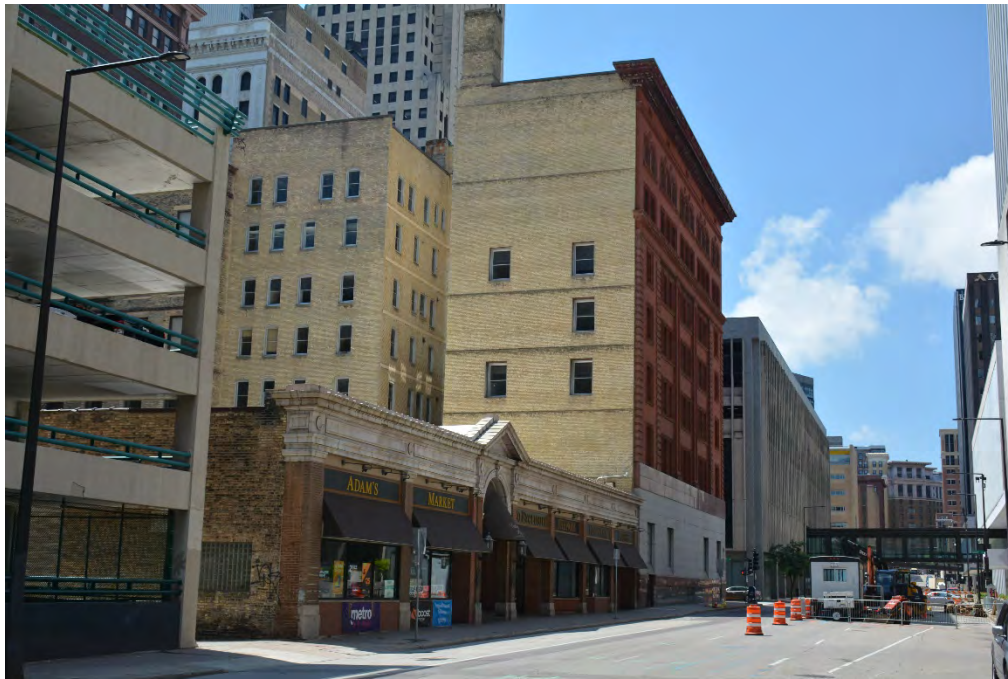
Figure 45. Endicott Arcade Addition, facing southwest with Manhattan Building and 5th Street / Robert Street Station site in the distance
