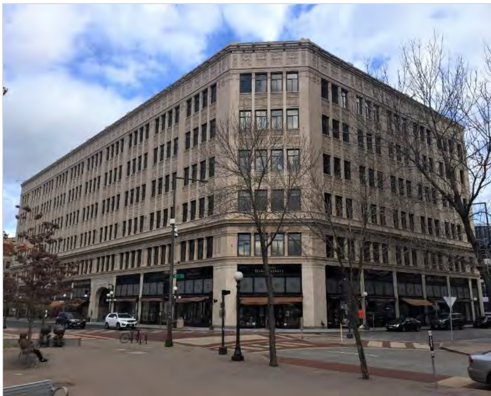
Figure 67. Hamm Building, facing north-northeast
