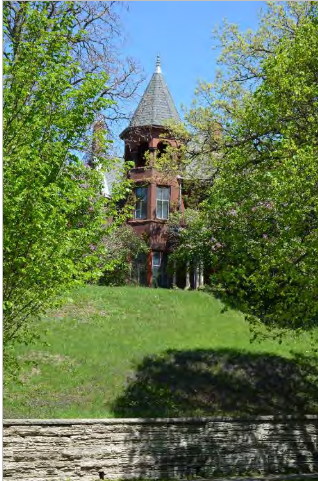
Figure 21. Giesen-Hauser House, facing northeast
