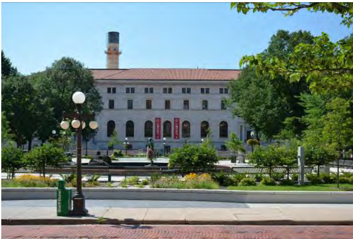
Figure 62. Saint Paul Public Library / James J. Hill Reference Library, facing south
