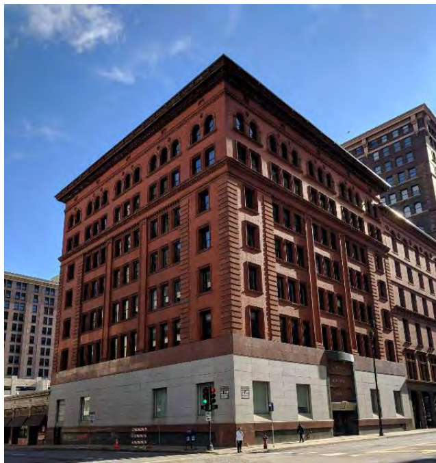
Figure 49. Manhattan Building, facing east
