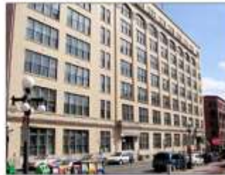
Finch, Van Slyck & McConville Building
