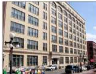
Finch, Van Slyck & McConville Building
