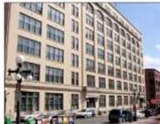
Finch, Van Slyck & McConville Building
