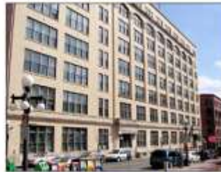
Finch, Van Slyck & McConville Building
