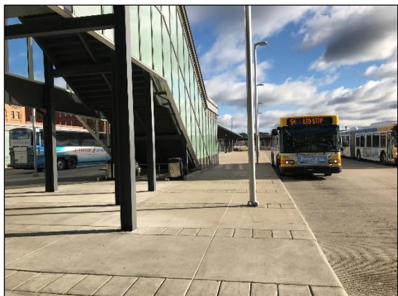
FIGURE 4.5-5: EXISTING UNION DEPOT BUS DECK
