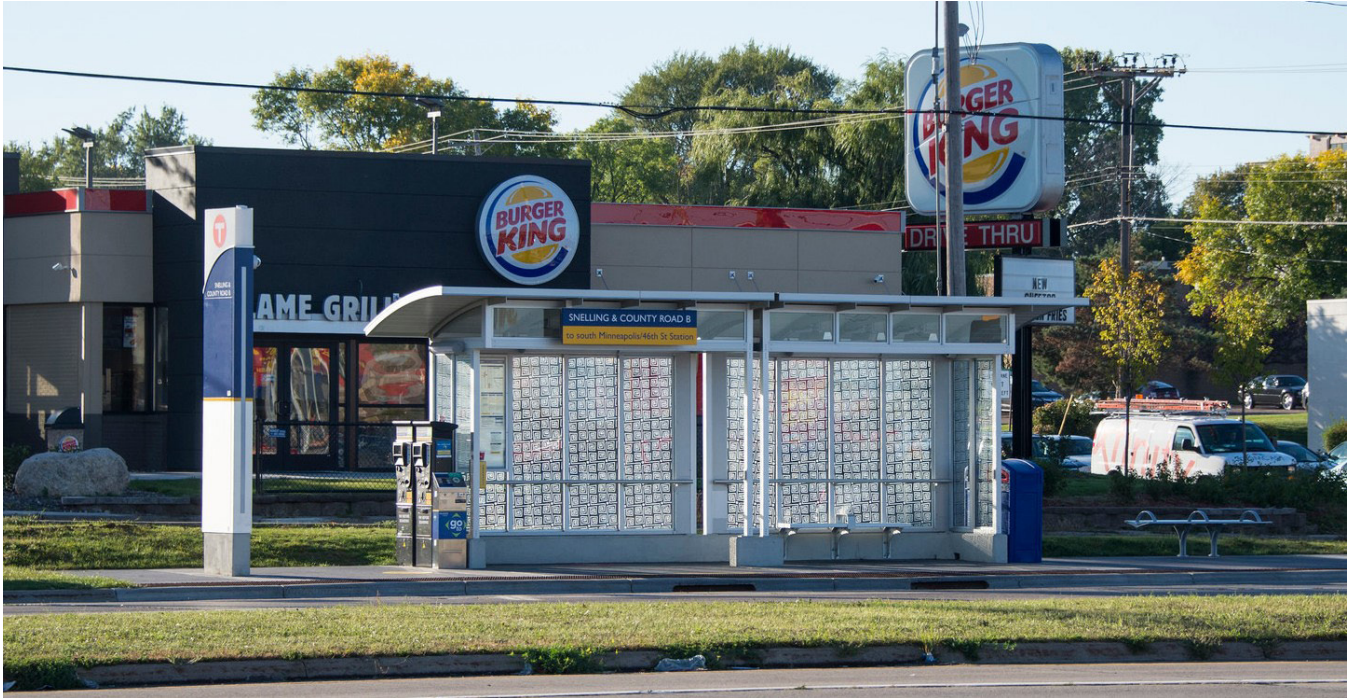
Figure 12: Medium shelter on the A Line, Snelling & County Road B station
